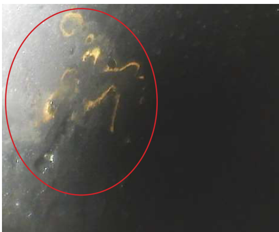
Figure 5: APR Tube #120, 57.2% wall loss (pitting) at 8.15m
